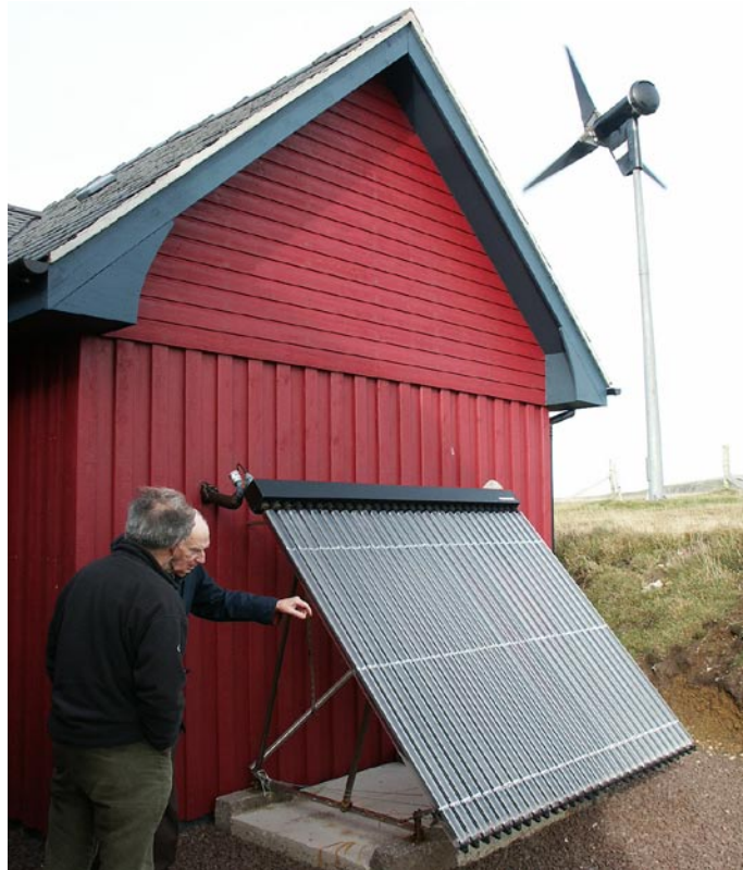
A windmill and solar water panels provide electricity and heat for a house on Fair Isle, near Shetland
