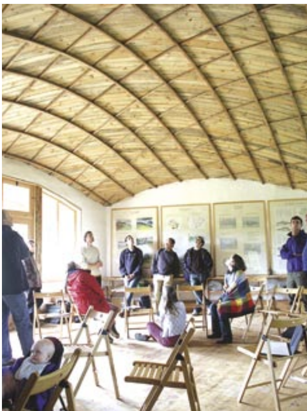
This shows a gridshell roof construction which uses a very small amount of timber to form a substantial span. The gridshell is braced by the overlayers of timber boarding.
